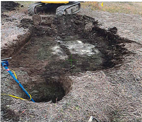
Above - Excavation of gas leak area – white area indicating gas leak
